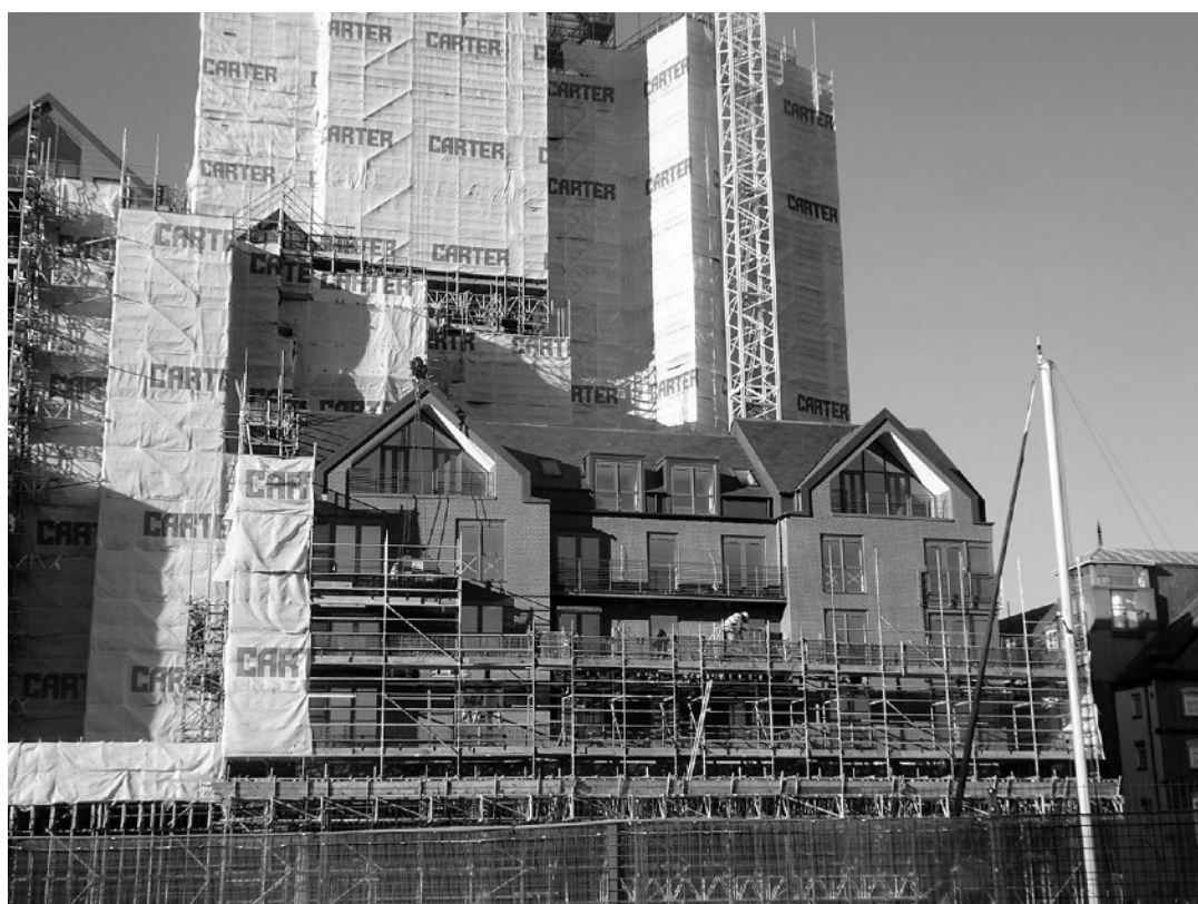
The Winerack scaffolding coming down, February 2019.
