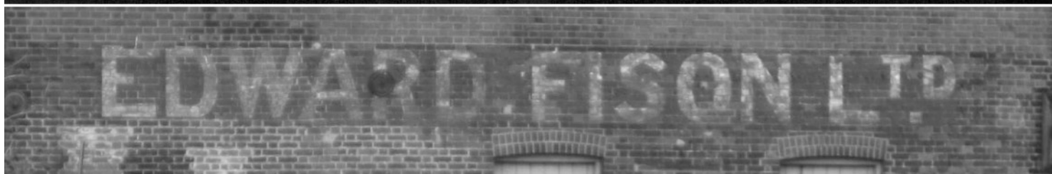
Top: The Edward Fison Ltd. sign (with bonus 'Webster's Trade Yard' lettering – now gone) photographed in 2000 from the Island site. The building fronts Dock Street in Over Stoke. Below: the sign has benefited from weathering, the characters more pronounced by 2012. [Photographs from the Ipswich Historic Lettering website.]
