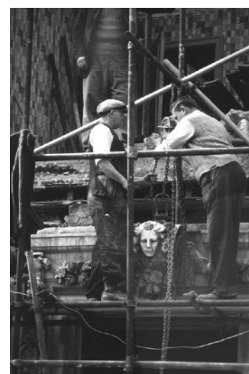
8 Princes Street, May 1966 Demolition, removal of doorway sculpture
