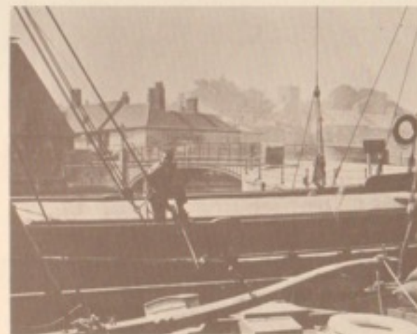
The old Stoke Bridge, built by Ransome's in 1818.
