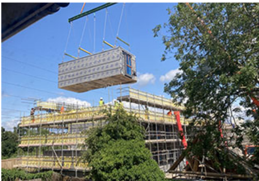
L&G modular units being dismantled at Bristol site earlier this year because of foundations problems.
